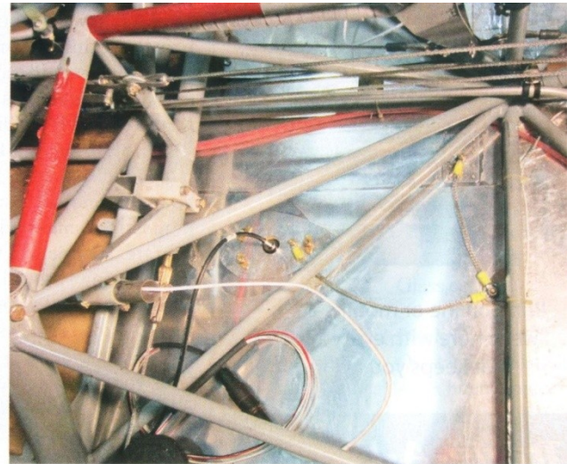
New ground planes and bonding straps, shown with the GlaStar seats removed.
